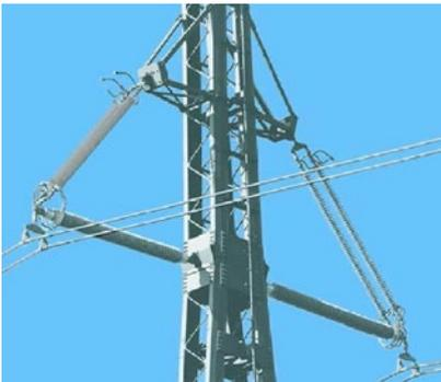
**Abb. 2.7** 420 kV Isoliertraverse
